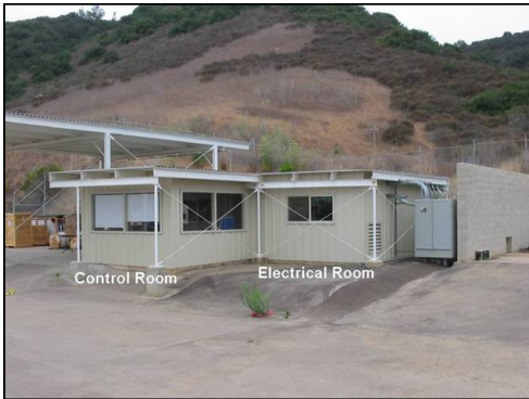
Figure 4. Test track control and electrical rooms.
