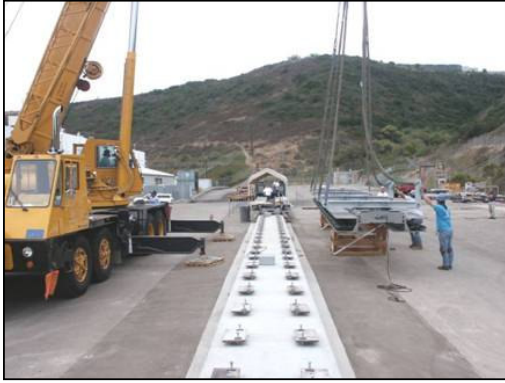
Figure 2. Installation of a 15-meter guideway module.
