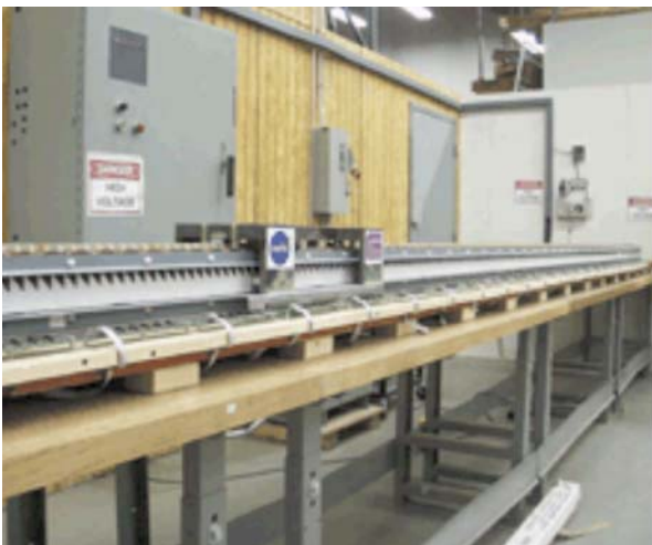
A scale model of the linear induction track at Foster-Miller. Preliminary tests of its maglev launch system were conducted with a 40-foot-long synchronous motor.
